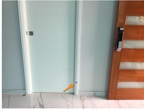
Ground Floor Front Right
