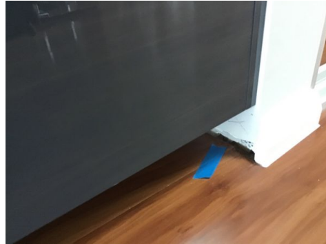
1st Floor hall
