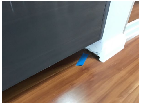
1st Floor skirt missing
