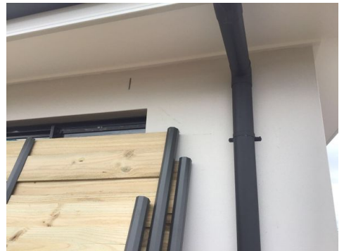
Ground Floor Rear
