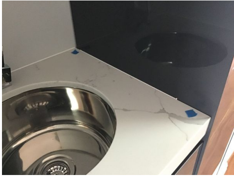
1st Floor basin
