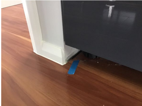
1st Floor hall
