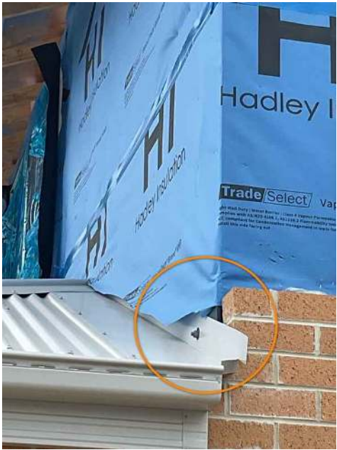
Front. Lap sarking over flashing
