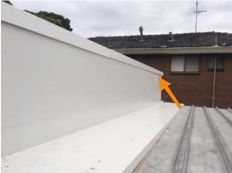
Not tucked under capping
