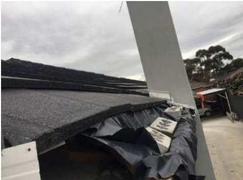
Not tucked under capping
