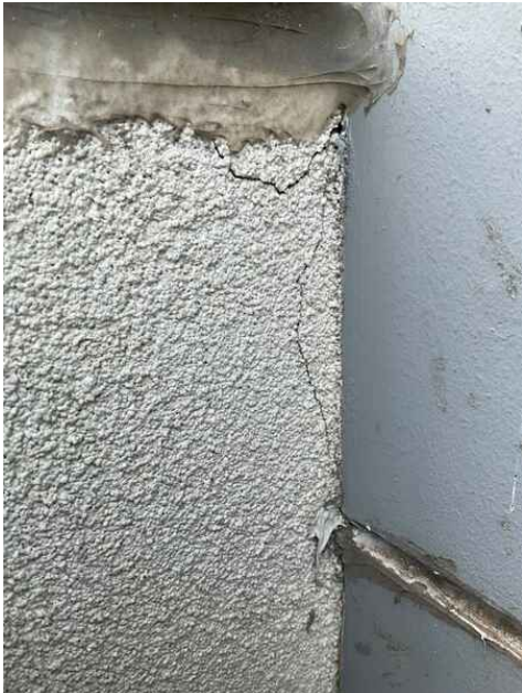
Render crack over garage - No.2
