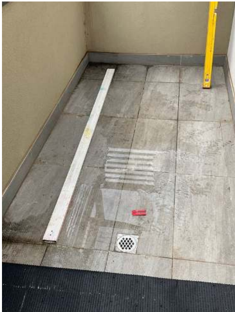
Water ponding to balcony above the water stain area
