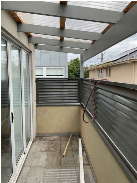
Roof over balcony.
