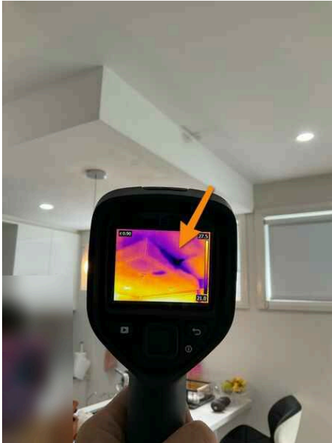
Moisture increased substantially with time after hose test
