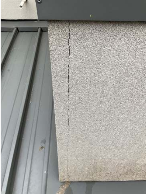
End of flashing is not sealed.
