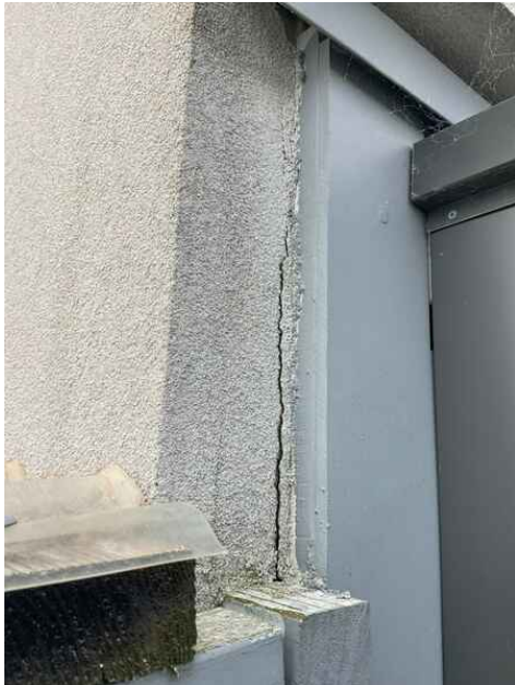
Render crack over garage - No.1
