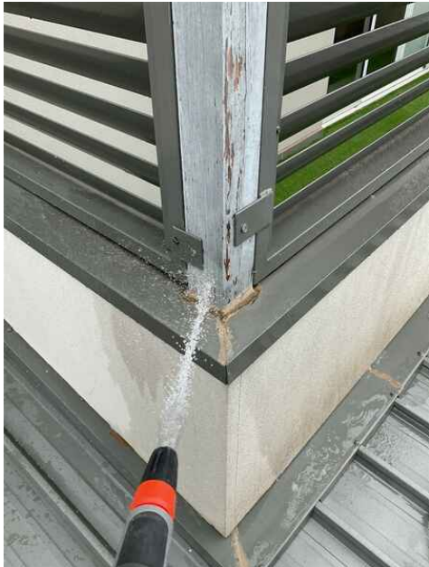
Hose test conducted to timber post above water stain in kitchen
