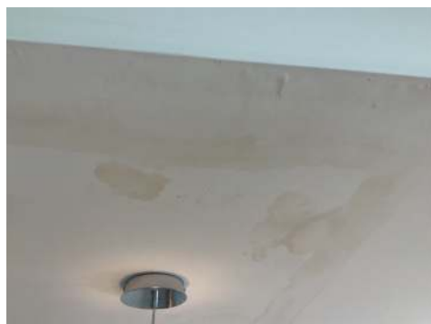
Water Stain and Mould to Kitchen Area
