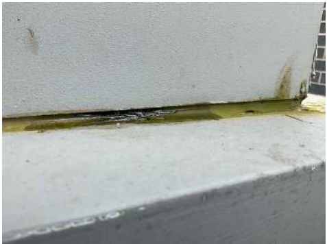
Sealing to matrix/flashing connection to be removed as per installation manual
