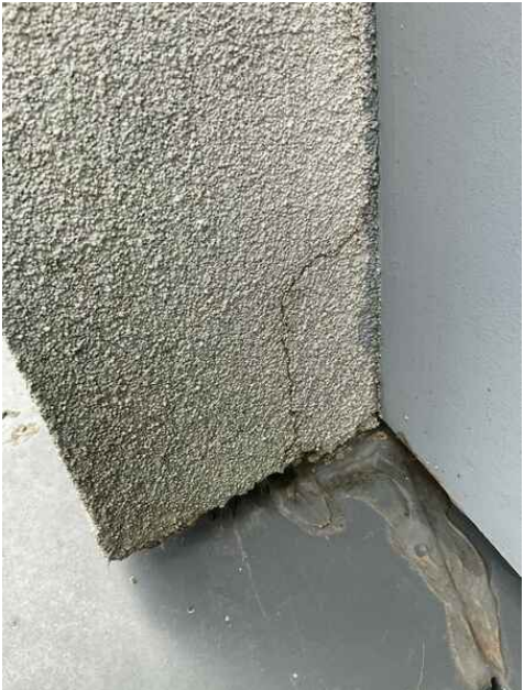
Render crack over garage - No.3
