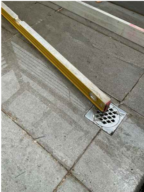
Using a 1200mm level, shows no fall at the drain
