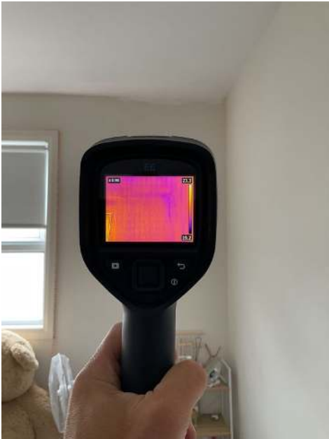
1st Floor bedroom
