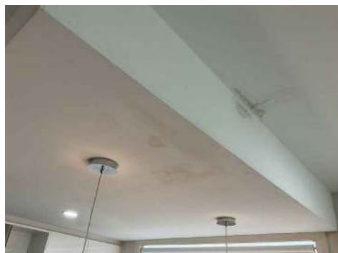
Water Stain and Mould to Kitchen Area
