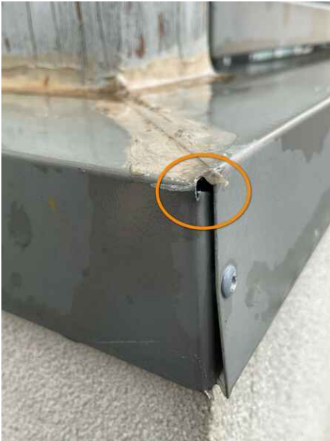
End of flashing is not sealed.
