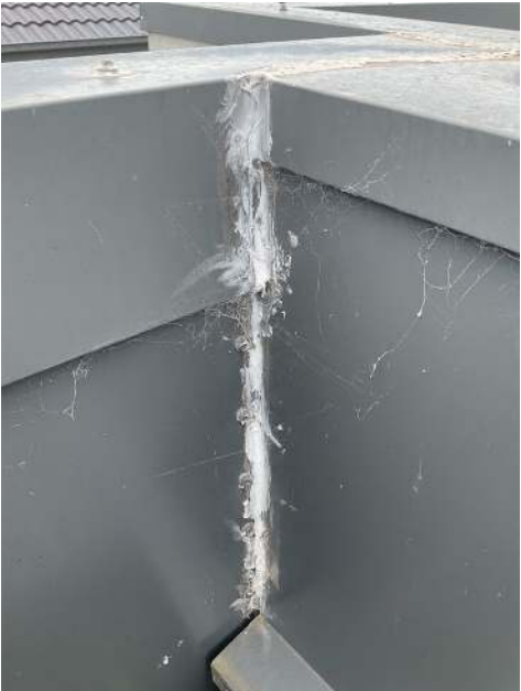
1st Floor roof
