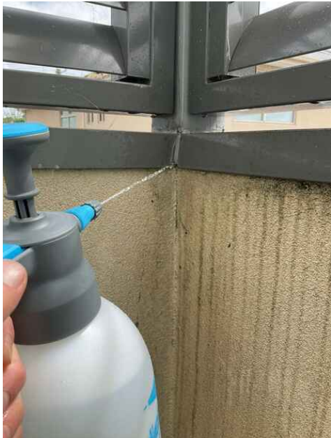
Hot water spray test to hole below metal capping to left corner of balcony
