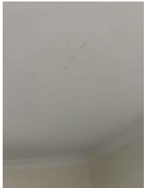
ceilings in the children's play bedroom appear to be letting go at the fixings this is consistent with water ingress from the roof space
