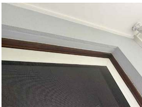
Upper-level window head corner with insect screen — head trim / reveal detail relevant to the window head-flashing assessment (Items 13–18).
