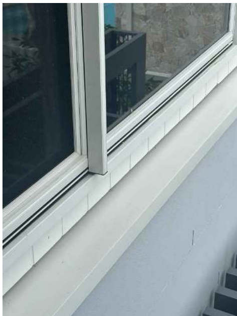
Upper-level window jamb / sill corner with the adjoining canal reflected — window perimeter and sill meeting the cladding (coastal exposure context).
