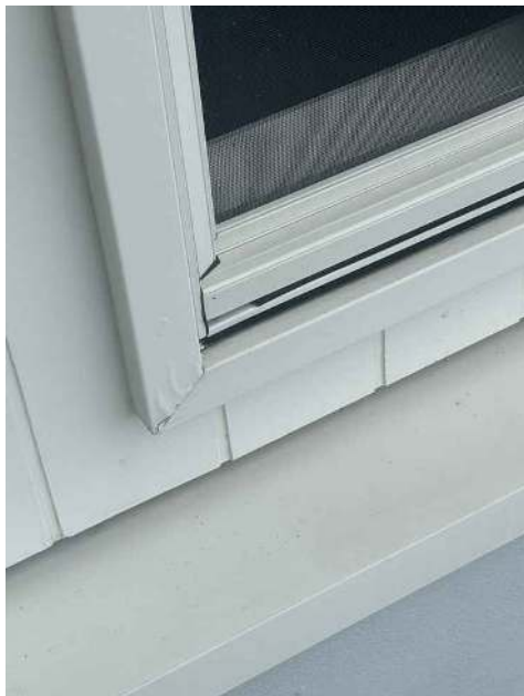
Upper-level window jamb / sill corner with insect screen meeting the Axon cladding — window perimeter and sill detailing relevant to the flashing assessment (Items 13–18).
