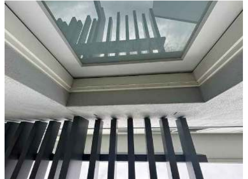
Window head beneath the pergola louvres with rendered reveals — alfresco area.
