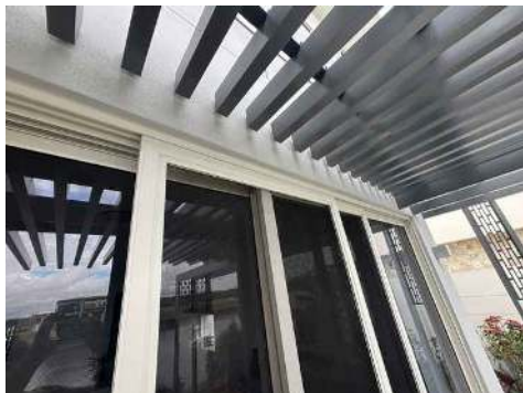
Alfresco sliding doors / glazing beneath the pergola louvres, with the outdoor area and canal beyond — coastal exposure context.
