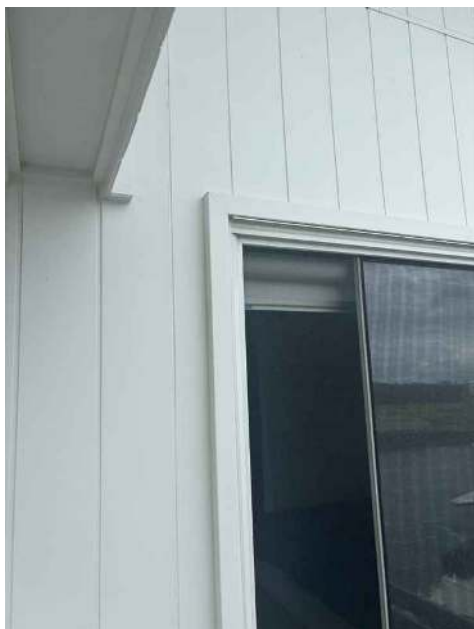
Upper-level window head / jamb in raking gable cladding — slim head trim with no projecting head flashing visible (Items 13–18).
