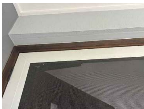
Alfresco / balcony area — window viewed beneath the pergola louvre structure with rendered reveals.
