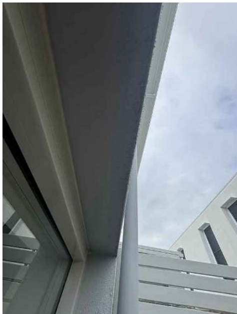
Eave / soffit and downpipe at a raking junction viewed against the sky — roof-edge and rainwater drainage detailing above the cladding.
