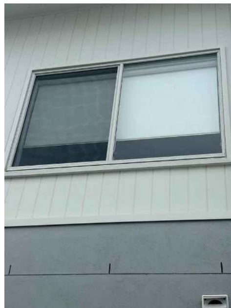
Upper-level sliding window with insect screen set in Axon cladding — head and surround relevant to the window flashing assessment (Items 13–18).
