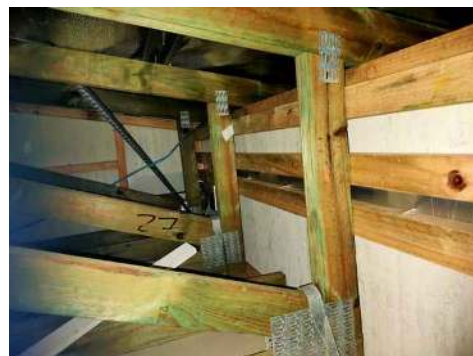
Roof-space structural framing — timber members with proprietary metal bracket connectors and bracing at the cladding wall.
