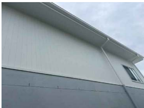
Gable-end elevation — Axon vertical-board cladding with eave above and a small upper window at right; cladding/render junction visible.
