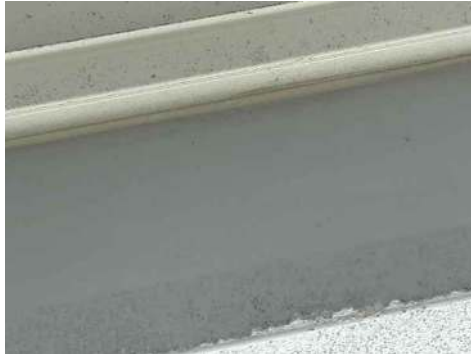
Eave / soffit and fascia underside — gutter and roof-edge detailing.
