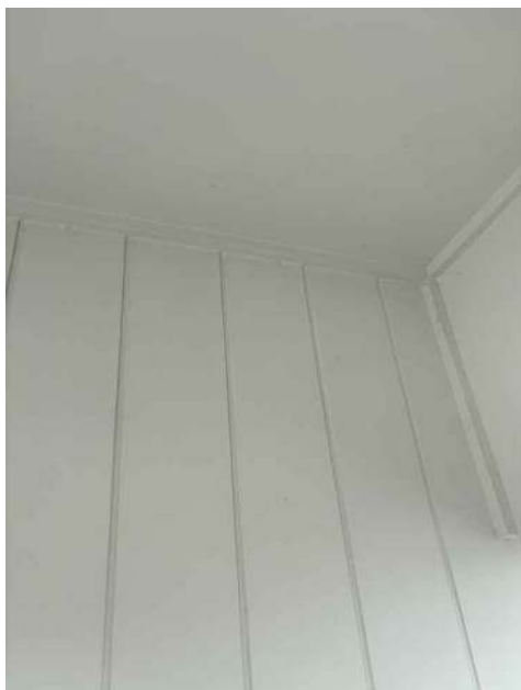
Eave / soffit underside and cladding return — representative of the upper-level eave and cladding terminations.
