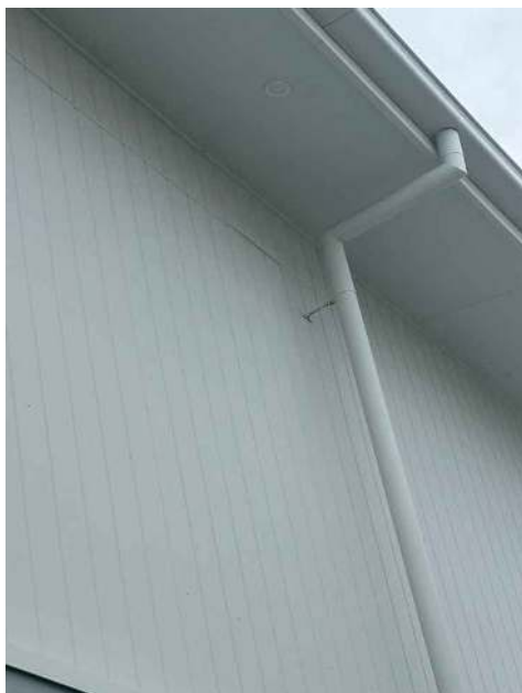
Eave / soffit underside with a downpipe running down the Axon cladding — rainwater downpipe and bracket location (Items 19–20).
