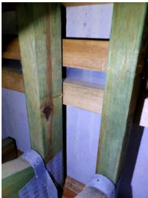
Roof-space framing — treated-pine studs/battens with a metal bracket connector and membrane behind; relevant to batten size/orientation and fixing into framing.
