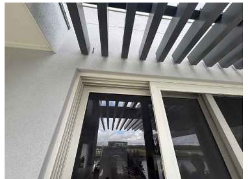
Upper-level sliding window with insect screen set in Axon cladding — head detailing relevant to the flashing assessment (Items 13-18).
