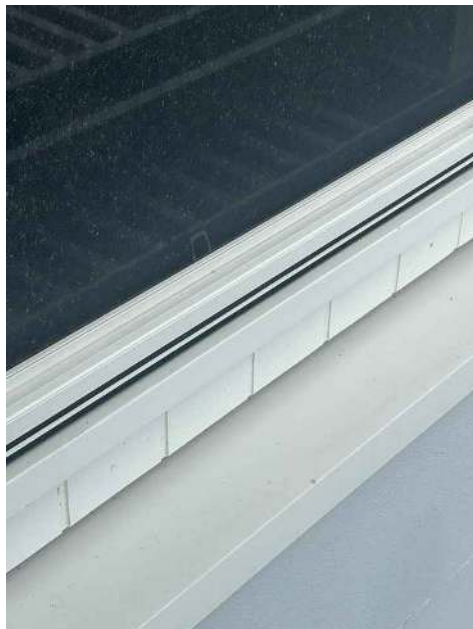
Upper-level window sill with insect screen — sill trim meeting the Axon cladding above the render; sill drainage detail relevant to the flashing assessment (Items 13–18).
