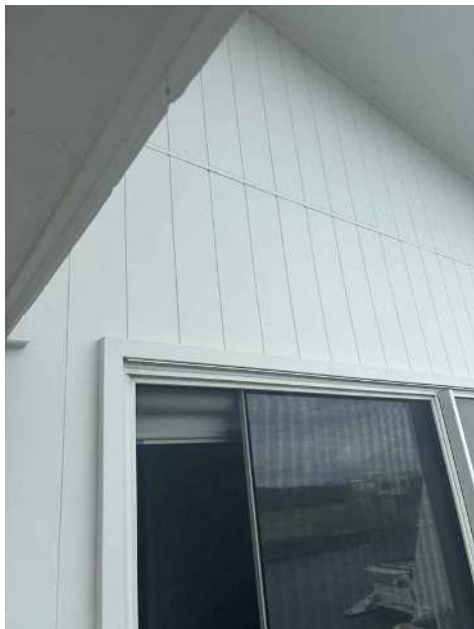
Raking gable cladding beneath the eave — Axon vertical boards at the gable; representative of the upper-level cladding terminations.
