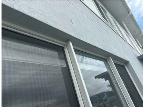
Alfresco glazing and screens beneath the pergola, canal beyond — coastal salt-water exposure context.
