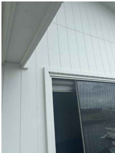
Raking gable cladding junction — Axon vertical boards meeting at the gable apex beneath the eave; membrane and flashing continuity significant at this junction.
