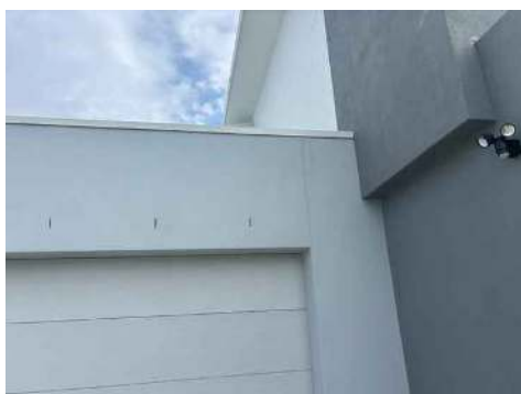
Rendered parapet / wall top with capping — external wall finish at the upper level. - no signs of moisture ingress from above.
