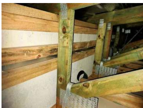
Roof-space framing — timber members fixed with metal strap / bracket connectors; load path and fixing into framing relevant to Items 9–11.
