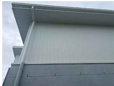
Gable-end upper level — Axon cladding with eave and gutter above and render below; horizontal joint line at the cladding/render junction.
