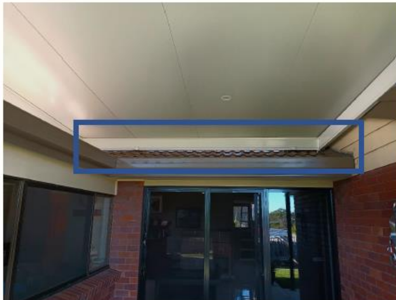
Photo No-6: Photo showing a lack of separation or clearance between the pergola and the house's roof.
