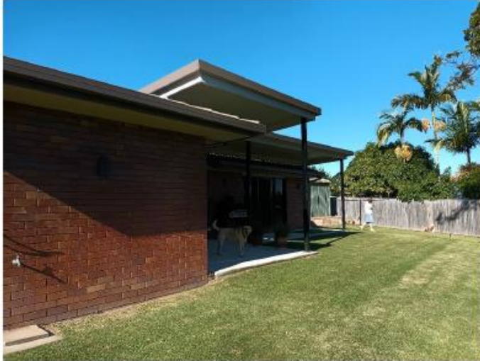
Photo No-6: Photo showing a lack of separation or clearance between the pergola and the house's roof.
