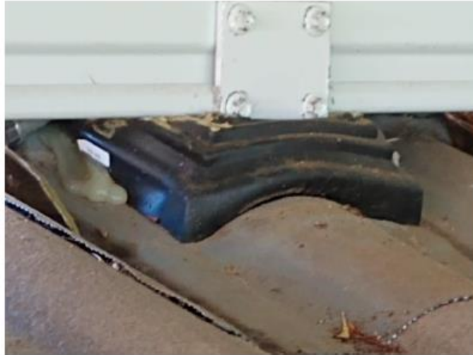
Photo No-8: Photo showing the pergola's improper roof pitch and how it directs water towards the house
