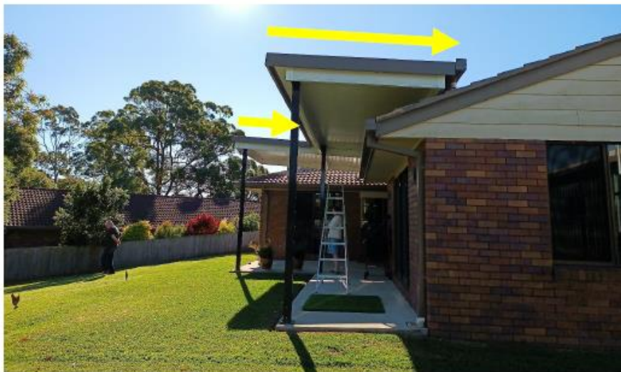
Photo No-8: Photo showing the pergola's improper roof pitch and how it directs water towards the house
