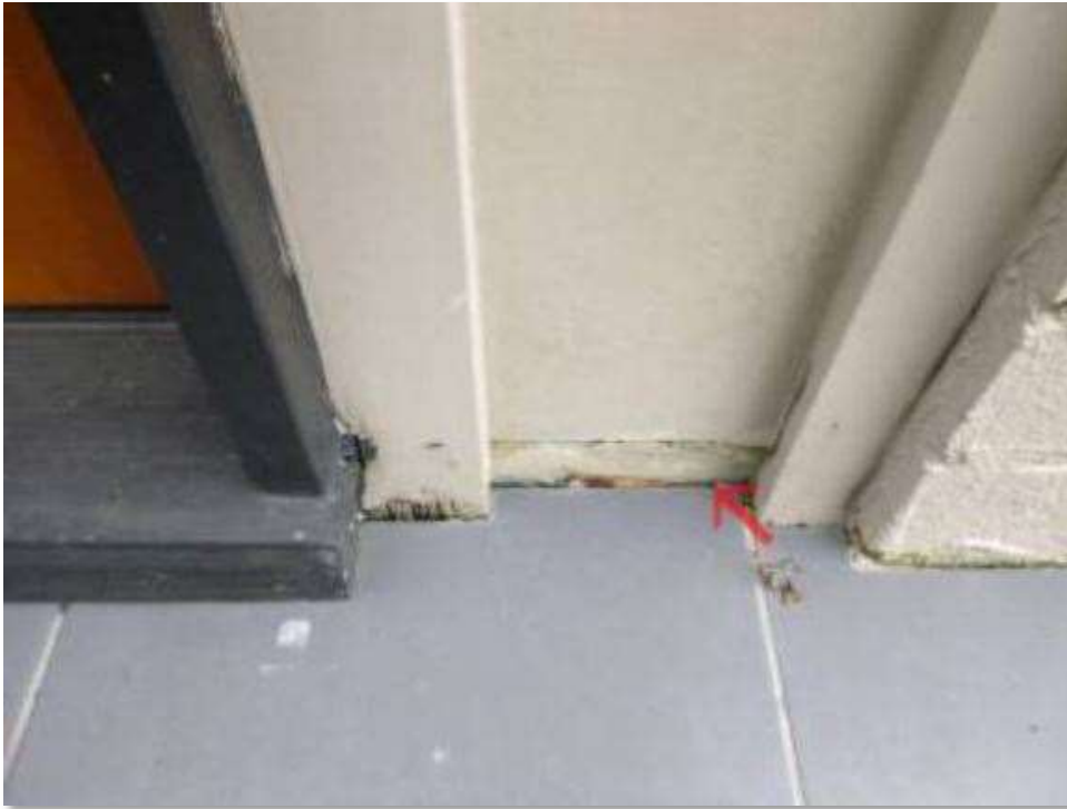
PHOTOGRAPH 5. CLADDING AND TIMBER BRIDGING TERMITE BARRIER
