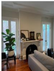
No cracks noted to the adjacent walls
